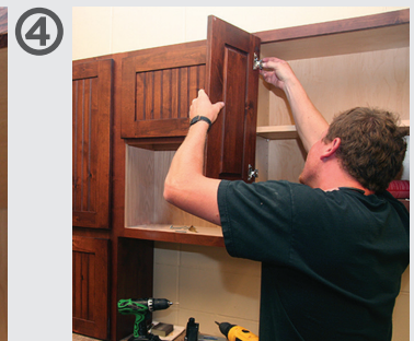
Install New Doors, Hinges, Drawers and Other Components
